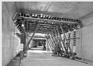
Tunnel formwork
