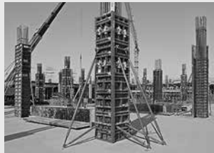
Column formwork
