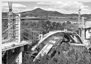
Bridge formwork
