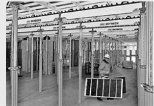
Slab formwork
