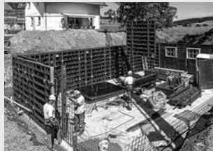
Wall formwork
