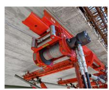
The units could be moved quickly thanks to an integrated cable winch.
