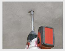
**Step 3**Screw in the refurbishment anchor by means of an impact wrench
