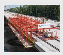
VGW Cantilevered Parapet Carriage
