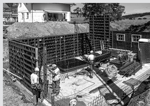
Wall formwork
