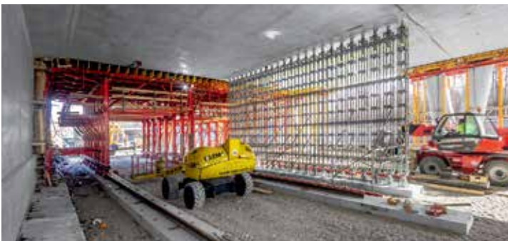
The modular VARIOKIT system can be adapted to suit different site conditions and to accommodate various areas of application.
