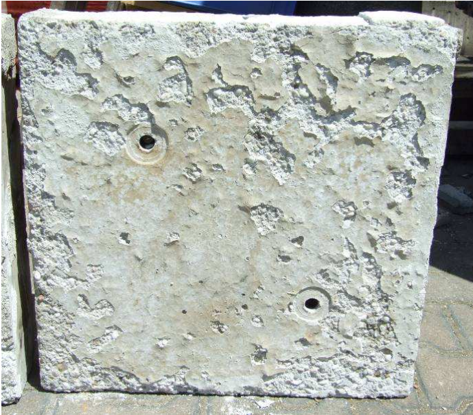
Photo 7 Exposed face after fire test
