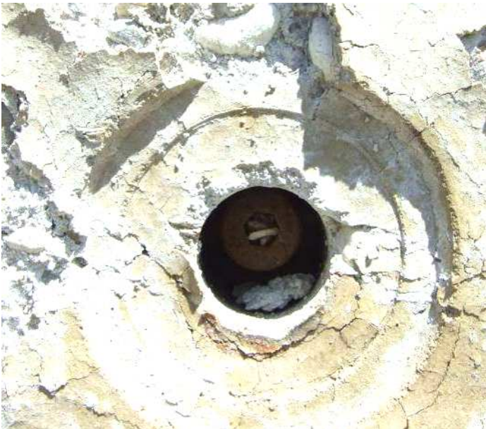
Photo 8 Screw plug "Schraubstopfen MX 15-50 OF-LS" Exposed face after fire test
