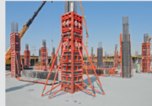
Column Formwork
