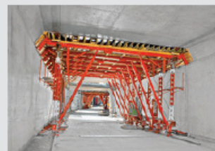
Tunnel Formwork
