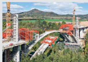
Bridge Formwork
