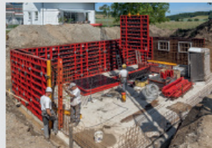
Wall Formwork
