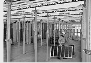
Slab Formwork
