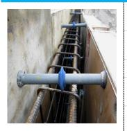
• Should be installed in the middle and over the outside of the formwork spacer with a concrete cover of minimum 100 mm.
