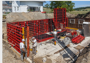
Wall Formwork
