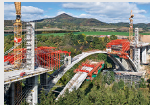
Bridge Formwork
