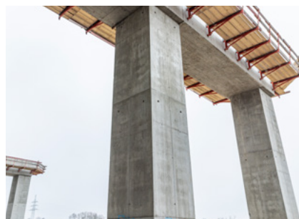
As working platforms, VGK Console Brackets provide safe and convenient working conditions.
