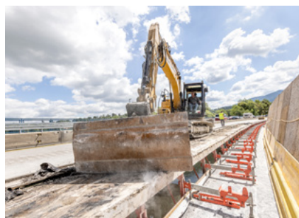
VGK Console Brackets ensure safety underneath the bridge and during work operations on the bridge.
