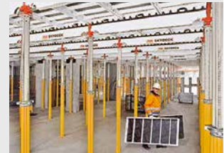
Slab Formwork
