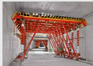
Tunnel Formwork
