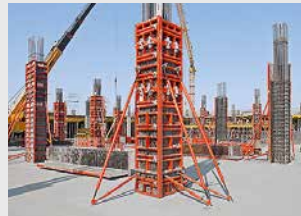
Column Formwork
