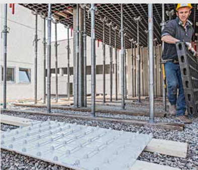
3. Installing the new formlining
