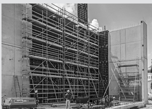
Working scaffolds construction
