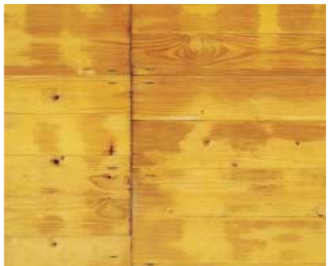
Forming the lining joint
