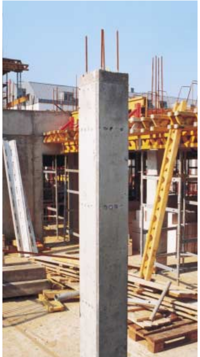
Columns with TRIO column formwork
