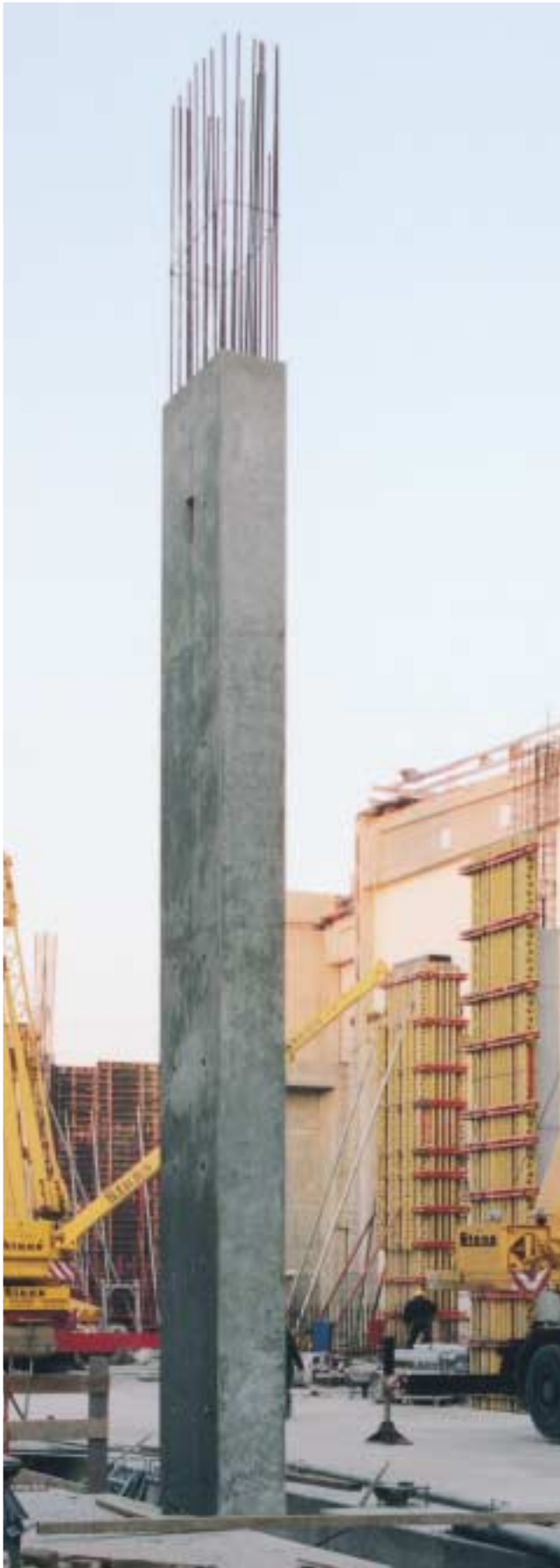
Columns with VARIO GT 24 column formwork
