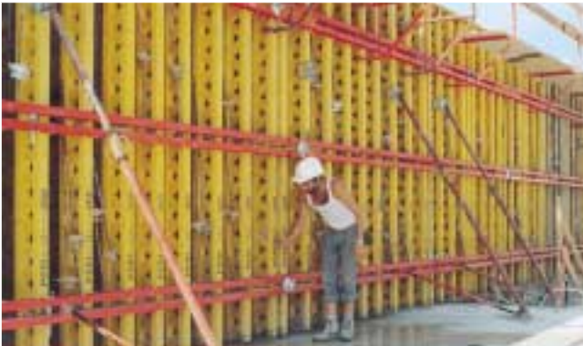
With VARIO Fair-Face Coupling installed
