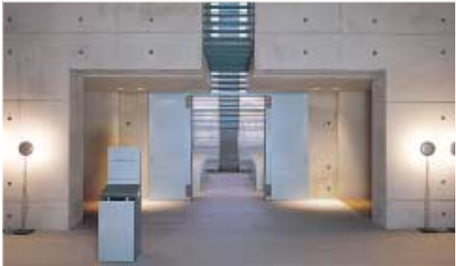
Watertight ties with cones and shadow joints Some formwork joints chamfered to form a concrete nib Ties and concrete nibs
