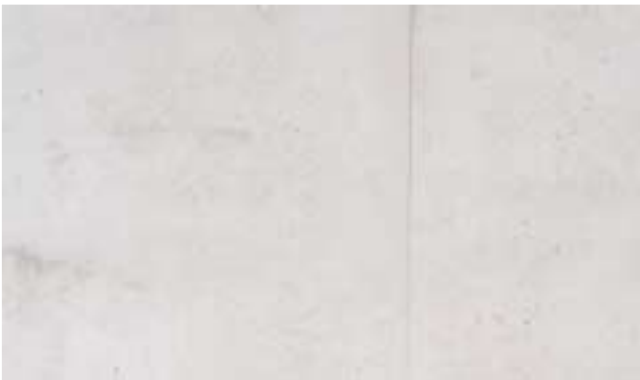
Unit joint in the concrete
