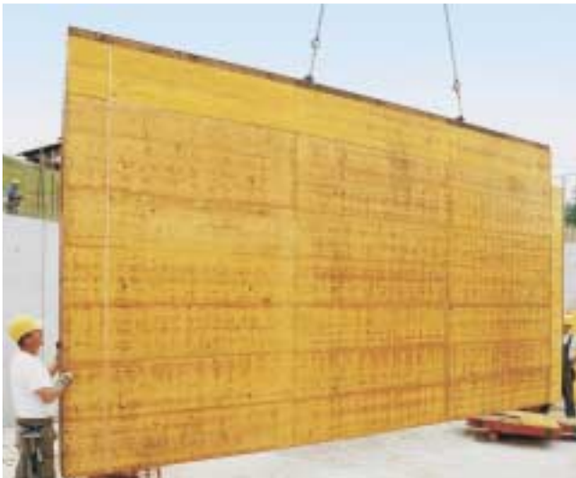
TRIO Structure units covered with 3-S panels
