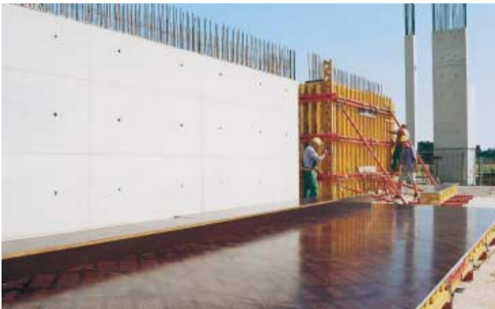
View of wall with joints and tie pattern
