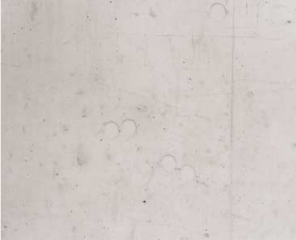
TRIO from the hire depot Formlining joint on a large panel
