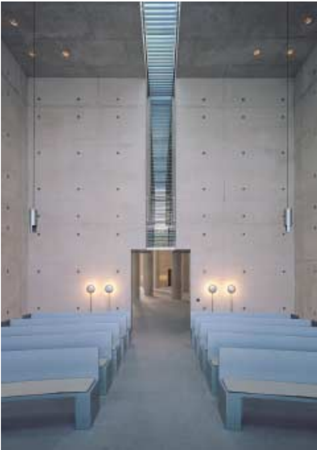
Watertight ties with cones and shadow joints Some formwork joints chamfered to form a concrete nib Ties and concrete nibs
