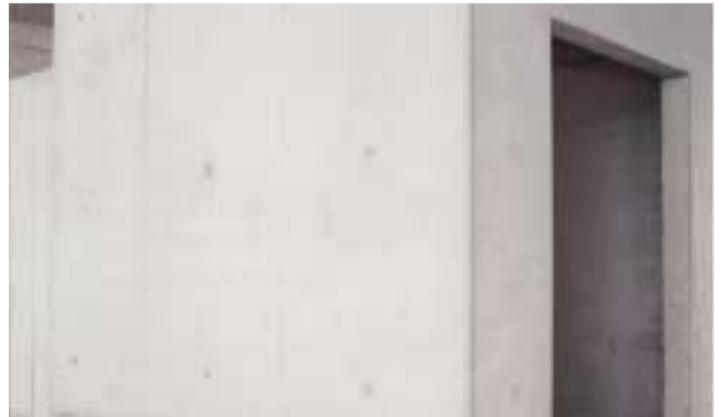
Picture of the unit and lining joints
