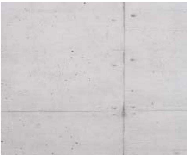
Picture of the concrete with unit and lining joints
