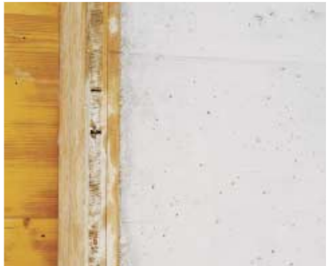
Forming of a door opening with chamfer strips
